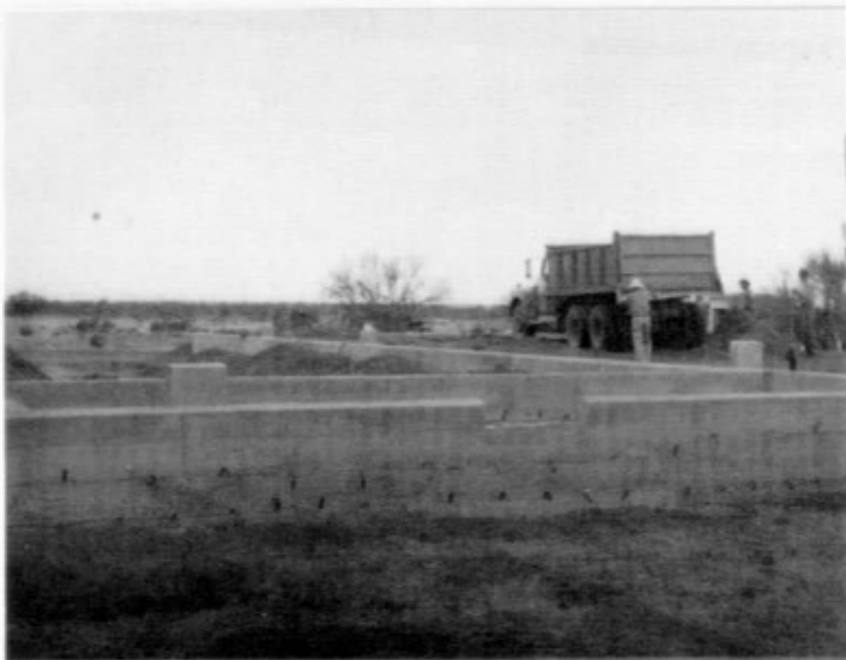
Man pushing truck over foundations.
