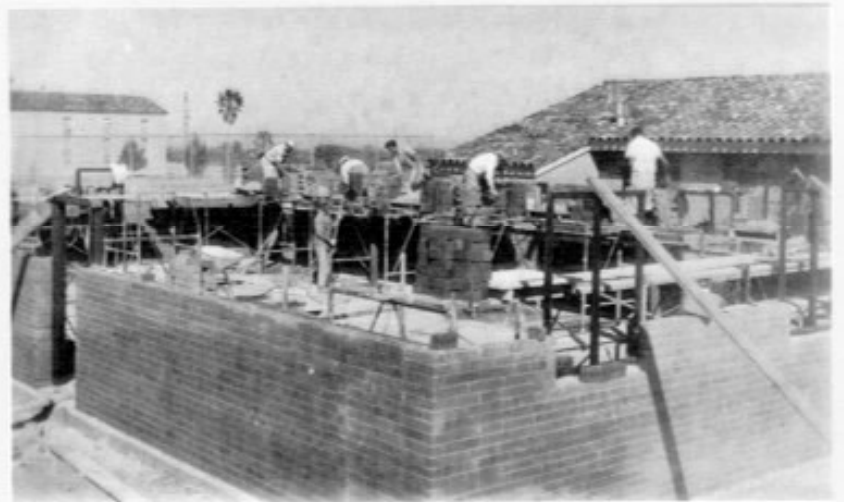
Construction of the activities building.
